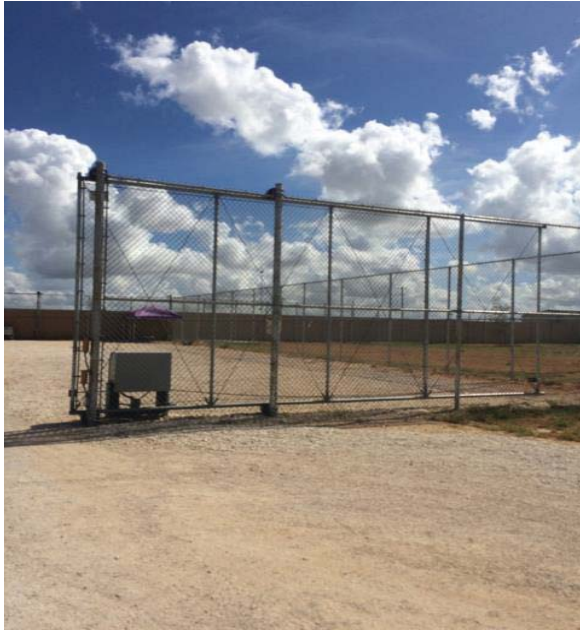
Figure 9. Security fence at Dilley Source: OIG
