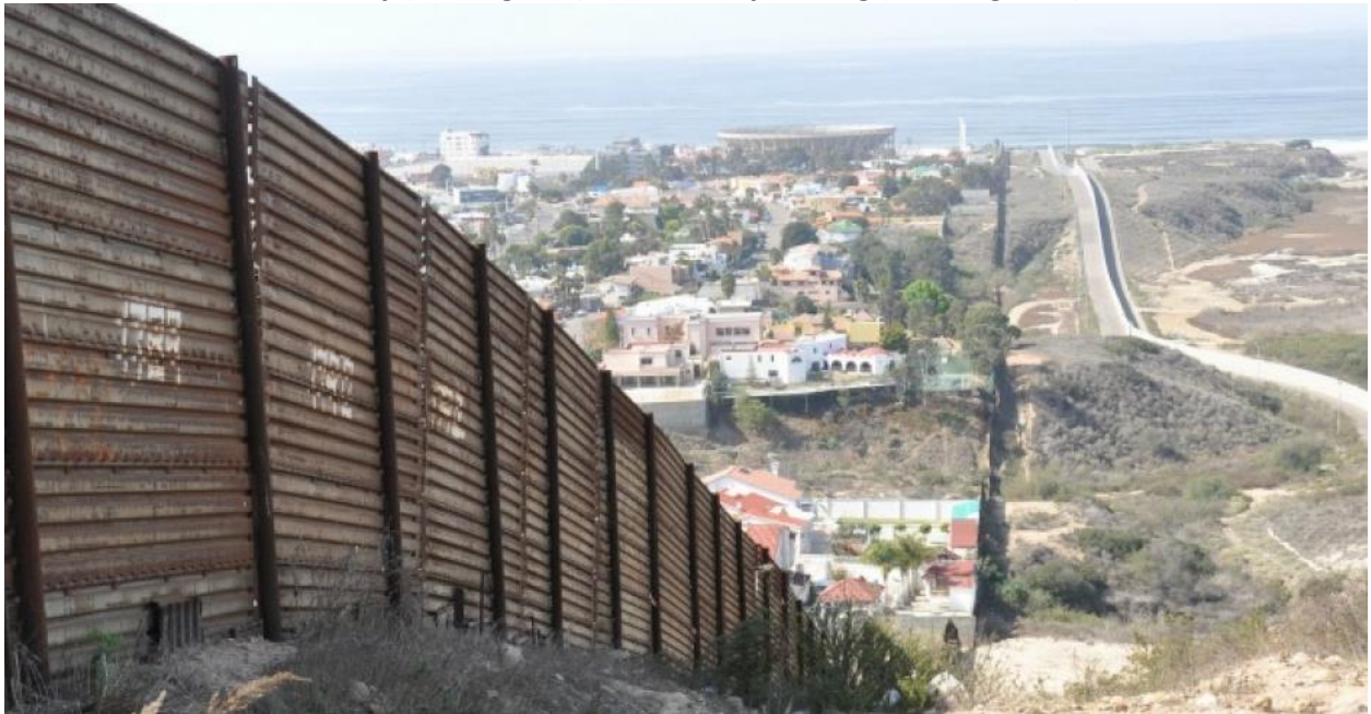
Primary (Landing Mat) & Secondary Fencing (San Diego, CA)
