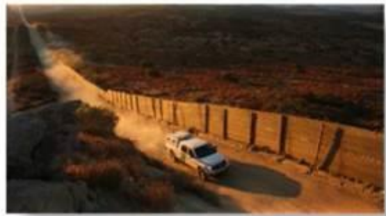
Pedestrian Fence: Landing Mat
