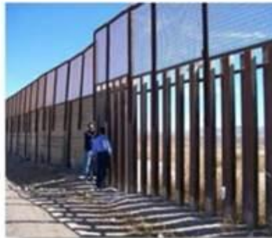
Pedestrian Fence: Slotted Steel with Mesh Panels
