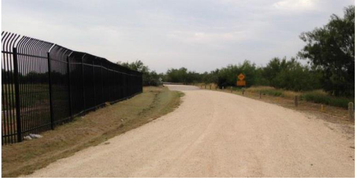
Primary Fencing (Laredo, TX) Collaboration between City of Laredo, Laredo College, Border Patrol
