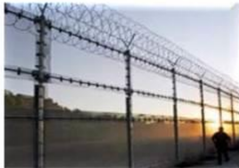
Vehicle Barrier - Normandy/Post on Rail (El Paso Sector)
