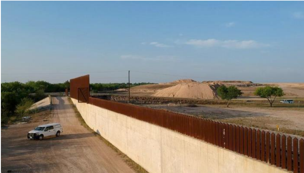
Levee Wall (Rio Grande Valley, TX)
