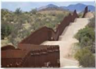
Pedestrian Fence: Bollard with Solid Steel Panel
