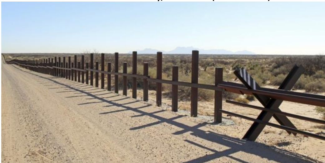
Vehicle Barrier - Normandy/Post on Rail (El Paso Sector)
