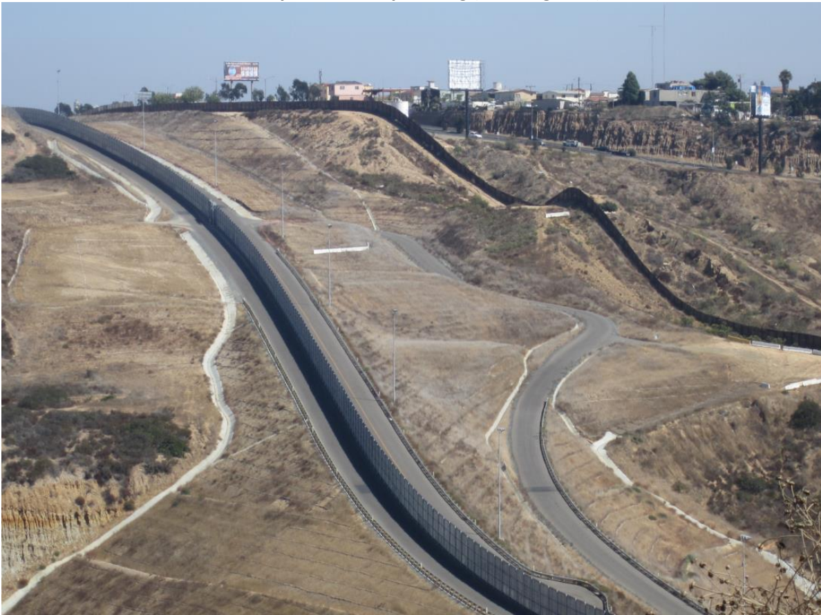
Primary & Secondary Fencing (San Diego, CA)
